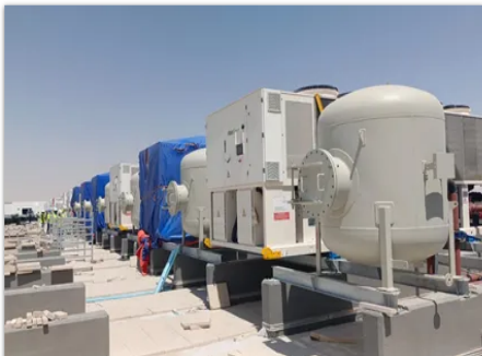
Chiller Installation Roof Top
