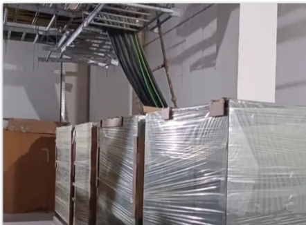
UPS Installation 1st Floor
