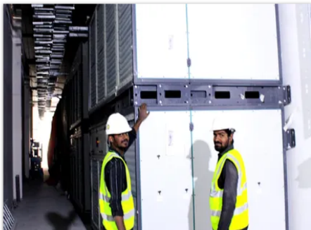
Fan Wall Unit 1st Floor
